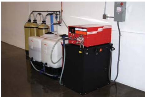
De-Ionizer Hot Pressure Wash System
